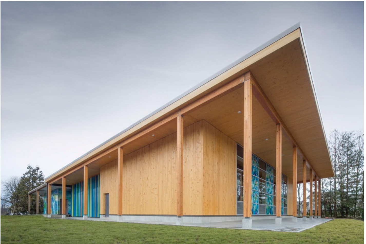
City of Richmond's ADEU energy centre
