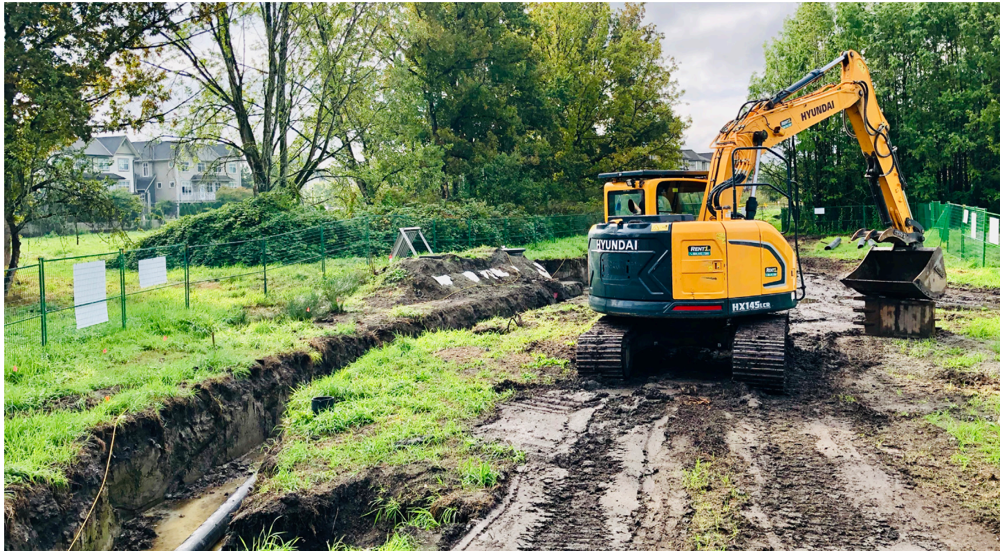
New distribution pipes being installed under Alexandra Park to allow for the future addition of new geo-exchange fields once the park is developed
