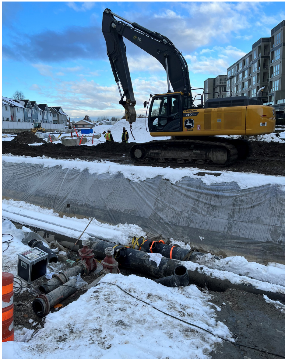
Implementing distribution piping in the ADEU.
